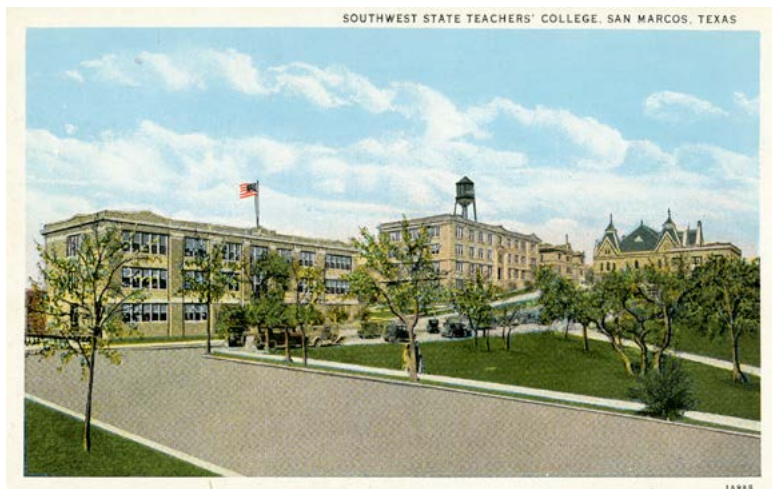
Early postcard of the quad, with the new Education Building on the left
